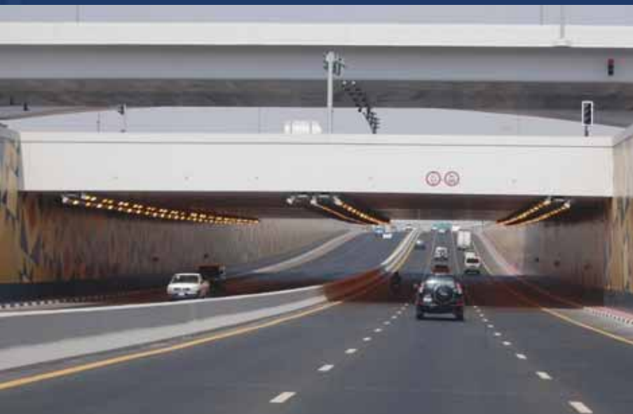
Left: Beirut Road Underpass Dubai
